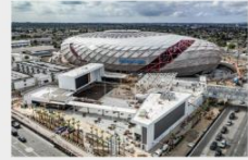
INTUIT DOME California; $130M+ project 18,000-seat arena -- home for the L.A. Clippers
