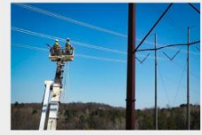
CENTRAL EAST ENERGY CONNECT New York; $300M+; 3 ½ year project Nearly 100 miles of 345kV transmission
