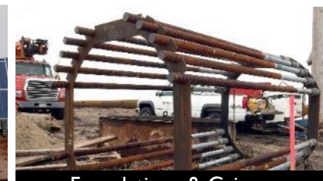
Foundations & Caissons and Directional Boring
