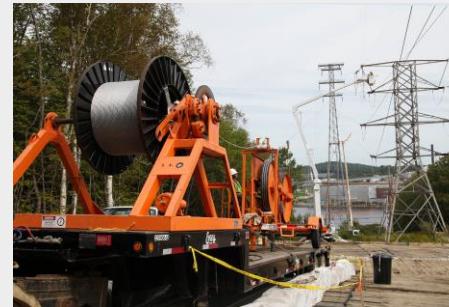
MAINE POWER RELIABILITY PROGRAM Maine; $200M+; 4-year project 210 miles of 345kV & 115kV transmission line
