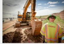
CENTRAL 70 TRANSPORTATION Colorado; $100M+; 4 ½ year project Electrical construction services
